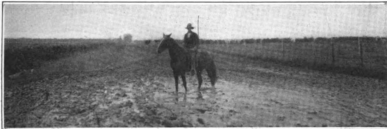
CHARACTERISTIC ROAD SCENE IN SOUTHERN ILLINOIS AFTER A HEAVY RAIN—BOTTOMLESS BLACK MUD AND STANDING WATER.
